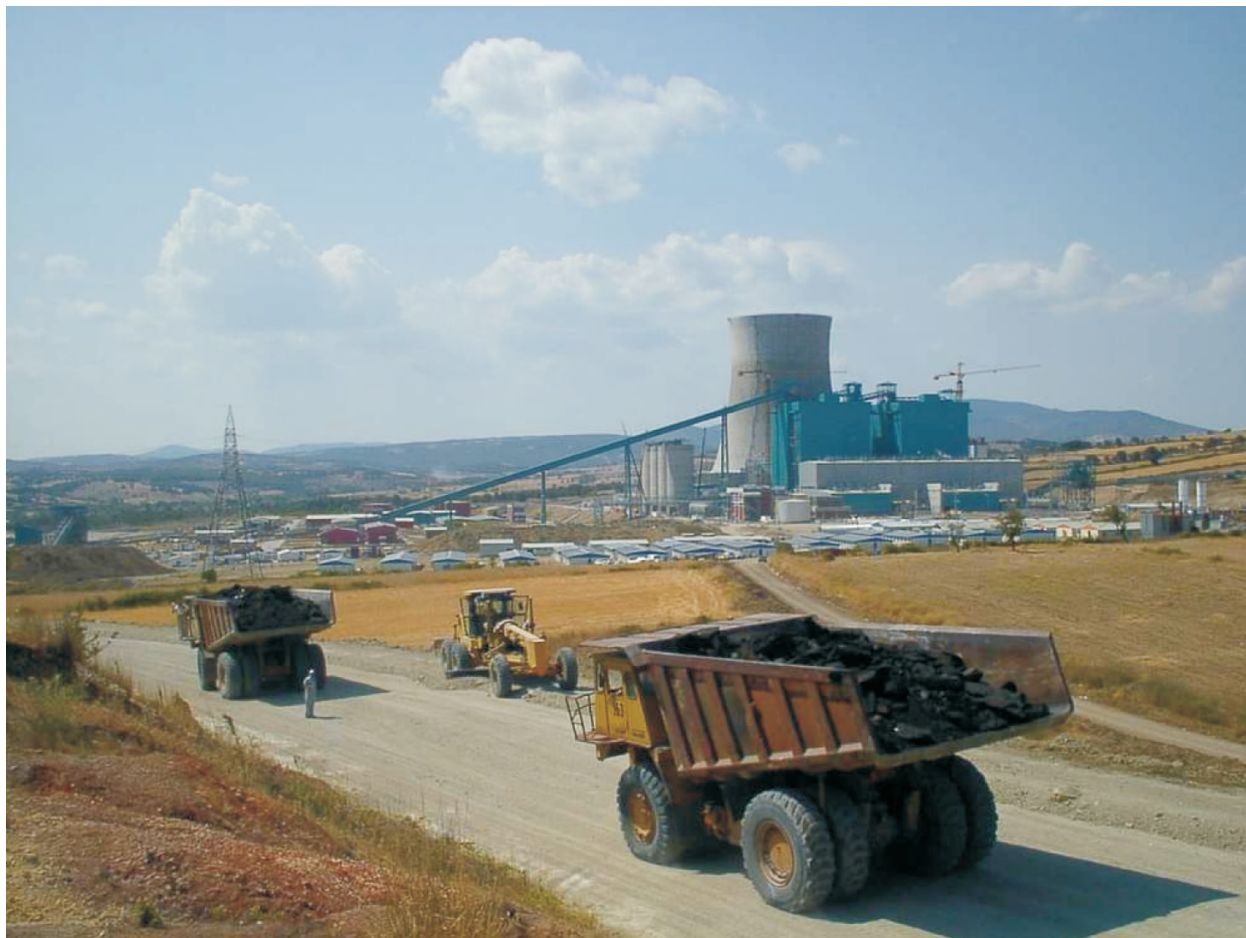
Figure 5. General view of the Çanakkale Çan thermal power plant.
