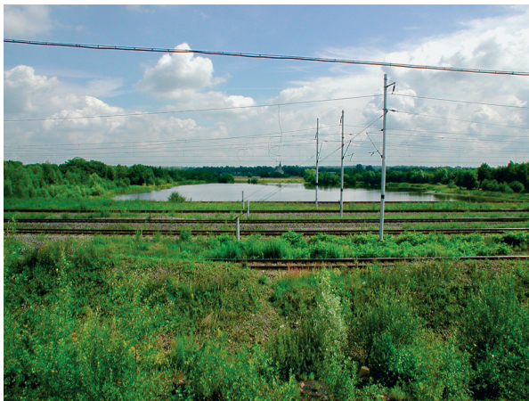
Figure 6. East part of Ostrava - Karviná coal field (2002; photo O. Mikulík). The main railway corridor from Ostrava (Czech Republic) to Žilina (Slovakia) crossing a large subsidence depression north of ČSM mine. This railway line is periodically renovated. Behind the railway line is a flooded subsidence depression.
