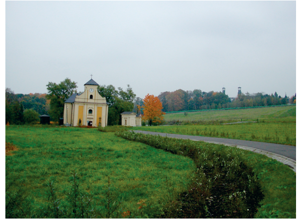
Figure 5. East part of Ostrava - Karviná coal field, Orlová town (2002; photo O. Mikulík). Church of St. Peter from Alcantary tilt towards road on account of the subsidence on the slope of protective pillar of Mine Doubrava.
