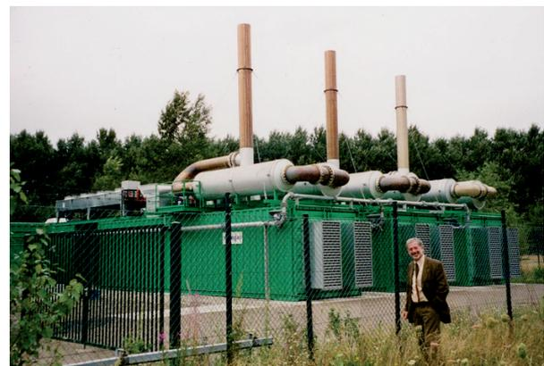
**Figure 6.** Abandoned coal mine gas (ACMM) production at Lünen Ruhr area, Germany. Gas (about 60%  $\text{CH}_4$ ) flows from the former shaft towards 3 gas-engine generators for production of electricity (total: 4MW).
