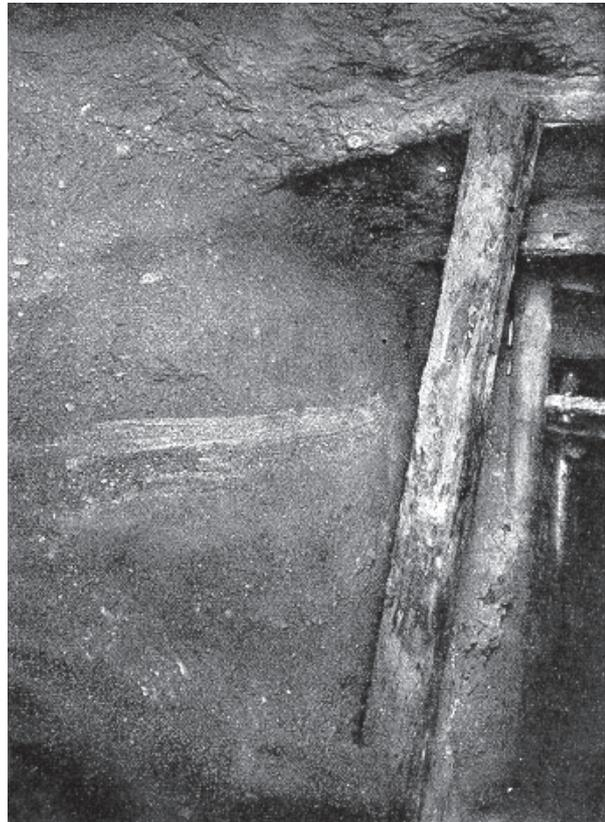
**Figure 4b.** Hydraulically stowed pillar.
