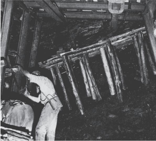
**Figure 3a.** Supporting the end of a main stone drift (inclined panel support in background).
