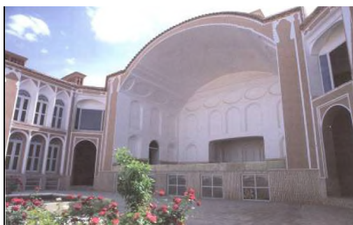
Figure 3: A view of Mortaz House
