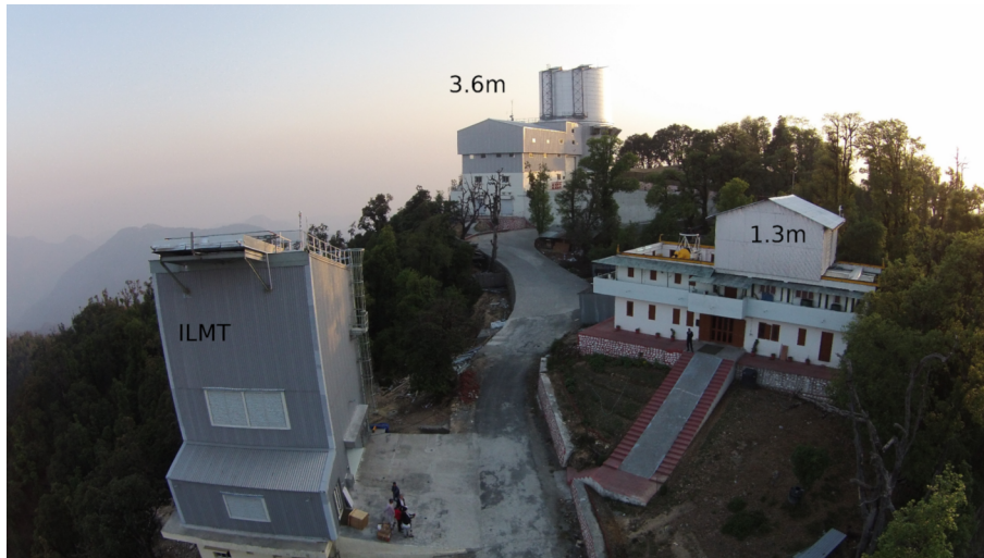
Figure 1: Aerial view of the Devasthal observatory located in the central Himalayan region of Nainital, Uttarakhand (Longitude = 79^{\circ}41'04'' E, Latitude = 29^{\circ}21'40'' N and Altitude = 2424 \pm 4 m). The housings of all the optical telescopes, marked with their sizes, are shown.
